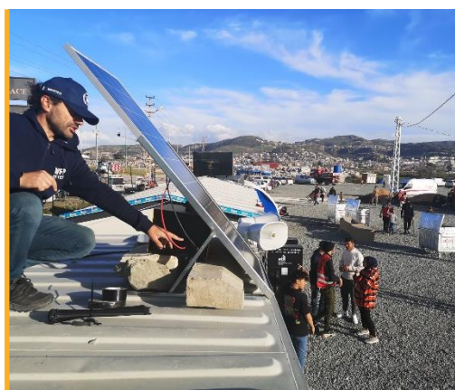
The ETS set up solar panels to support the charging station services for affected populations in temporary settlements in Hatay. Photo: WFP/ETS
