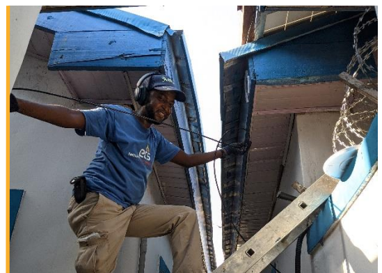
The ETS set up an access point to improve connectivity coverage at the humanitarian hub in Banki. Photo: WFP/ETS
