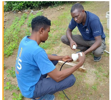
The ETS carries out maintenance to maximize services in Gwoza. Photo: WFP/ETS
