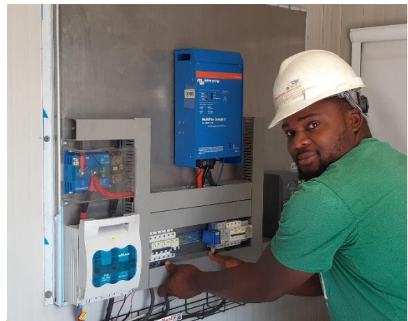
A contractor installs the ETS hybrid solar-power system in Monguno.
