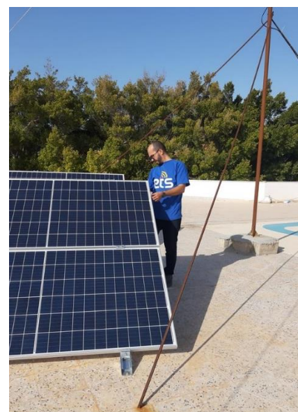
The back-up solar power system for the Security Operations Centre (SOC) is installed on the roof of the UN Hub in Benghazi.
