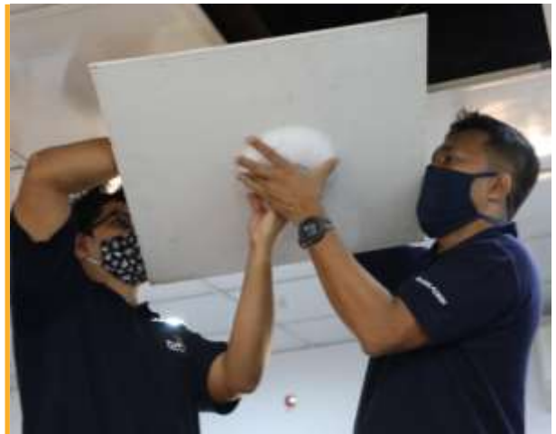
Installation of ETS data connectivity services in a new site, the ISCG office in Cox's Bazar. Photo: WFP/ETS
