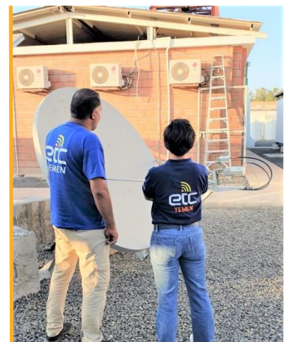
ETC and Head of WFP in Al Mokha visit the UN site to inspect the VSAT installation. Photo: WFP/ETC
