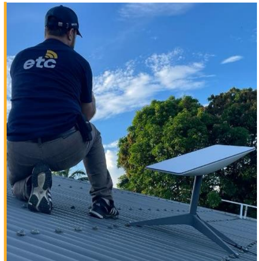
The ETC installing a Starlink satellite data terminal at Penama PEOC in Ambae. Photo: WFP/ETC
