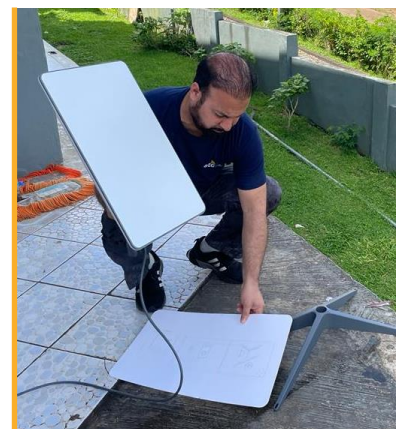
The ETC configured 10 Starlink satellite devices to link government responders on the islands to the mainland. Photo: WFP/ETC
