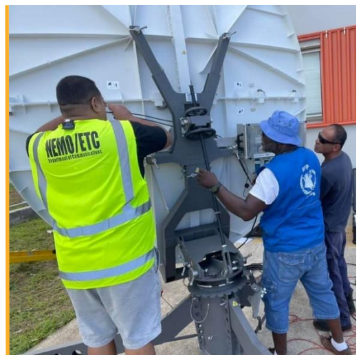
The ETC team installs the first emergency.lu VSAT for connectivity in Vava'u. Photo: MEIDECC/Pomaama Liu
