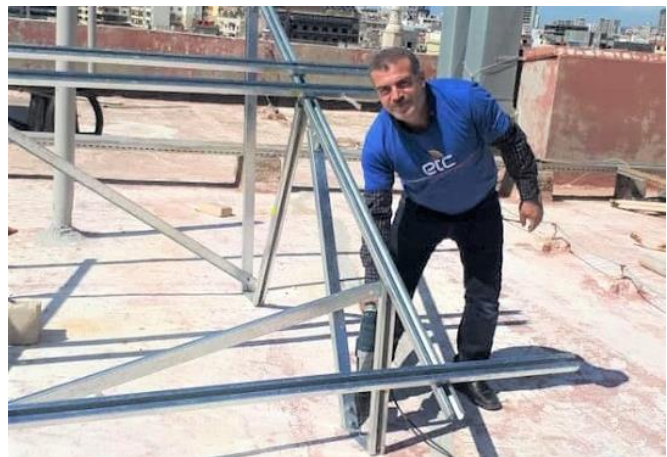
The ETC prepares to install the solar power solution in the Security Operations Centre (SOC) in Damascus.
