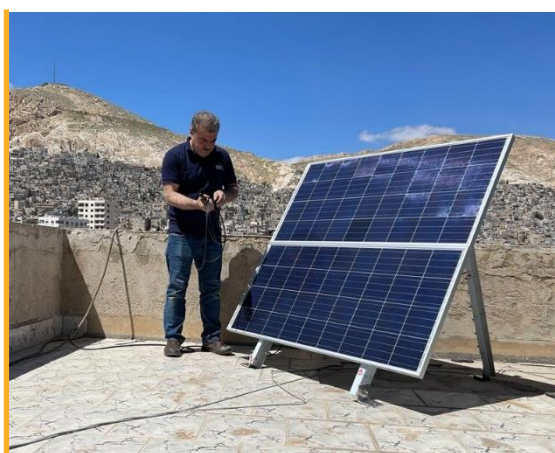
The ETC installs a dedicated solar power system for the VHF repeater at the UN hub in Damascus. Photo: WFP/ETC
