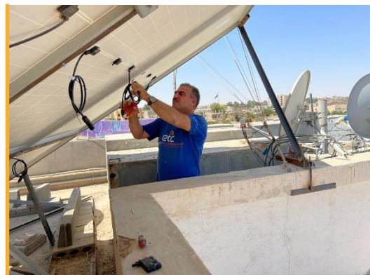
The ETC upgrades the capacity of the solar power system that supports the SOC and ETC data connectivity services in the UN hub in Deir Ez-Zor. Photo: WFP/ETC
