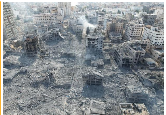
Buildings, telecommunications, and power infrastructure have been destroyed in Gaza due to the ongoing conflict. Photo: UNRWA.
