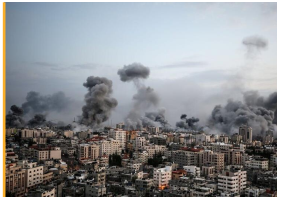
Buildings, telecommunications, and power infrastructure have been destroyed in Gaza due to the ongoing conflict. Photo: WFP/Ali Jadallah.
