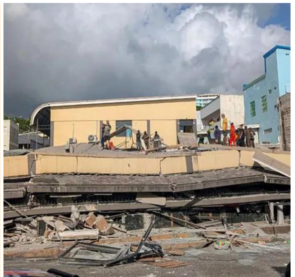
Multiple buildings collapse in Port Vila, Vanuatu due the impact of a 7.3 magnitude earthquake on 17 December. Photo credit: Getty Images
