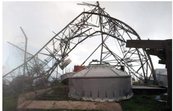
Telecommunications infrastructure in Vanuatu severely damaged by Cyclone Harold.
