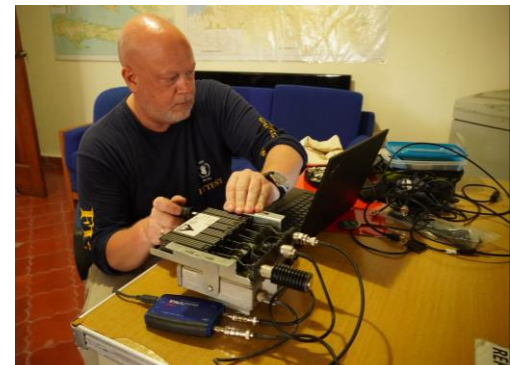
Photo: A WFP FITTEST technician prepares VHF repeater equipment for installation by emergency.lu and Ericsson Response in Jeremie.
