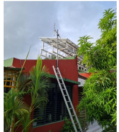
Photo: emergency.lu repeater installed by WFP FITTEST in Les Cayes
