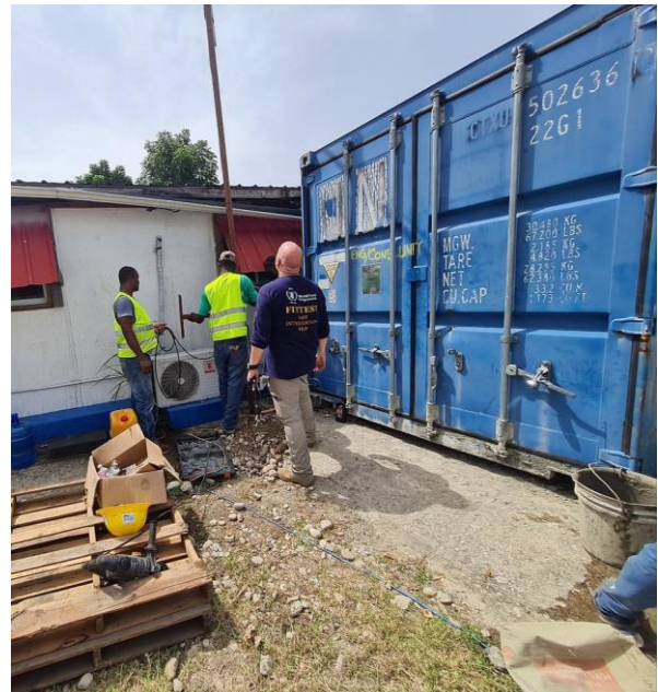
Photo: WFP FITTEST installs a VHF repeater in Les Cayes
