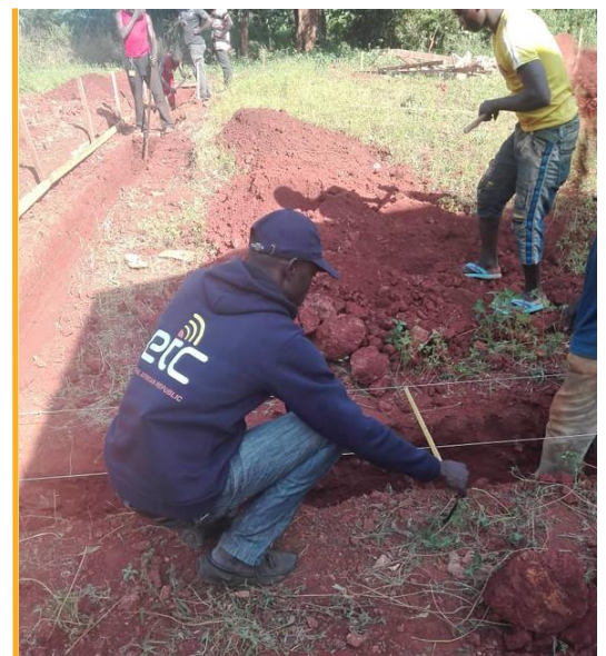
Construction work begins on the ETC Learning Centre and Cyber Café in Bangassou. Photo: WFP/ Nadege Ndassimba
