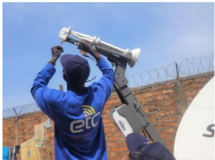
An ETC technician installs satellite equipment for data connectivity services in Zemio.
