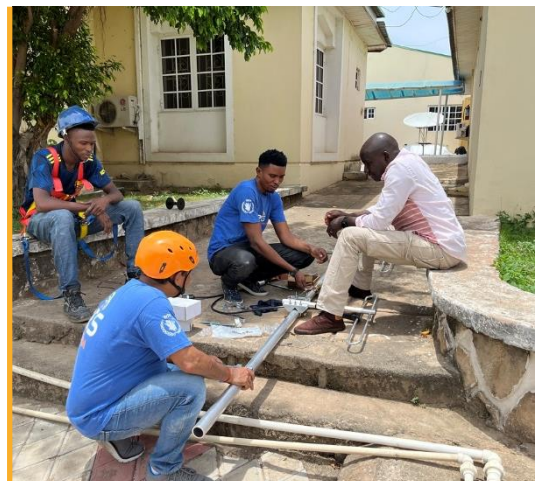
The ETS team regularly maintains and improves its services across 10 sites. Photo: WFP/ETS
