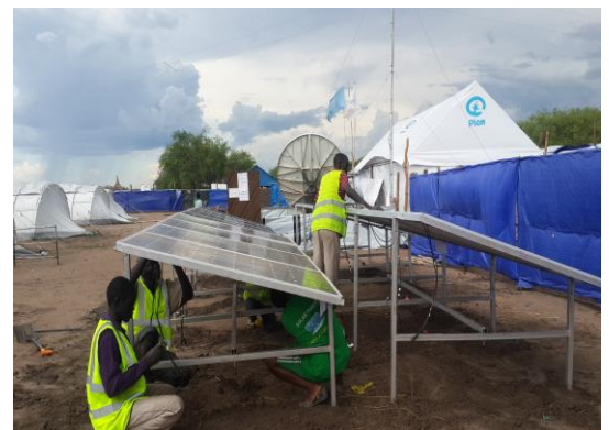
ETC installation of renewable solar energy solution at the Humanitarian Hub in Mingkaman, South Sudan
